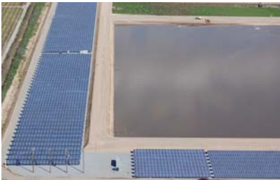
Elkhorn Dairy, 1MW single-axis trackers
