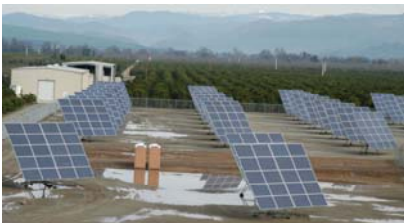
Venida Packing Co., 512kW dual-axis trackers
