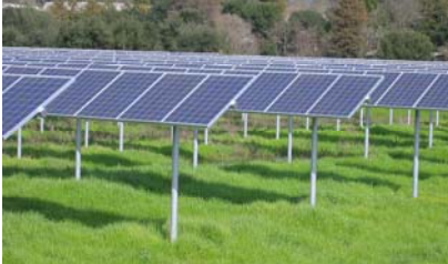
Napa Valley College, 1MW single-axis trackers
